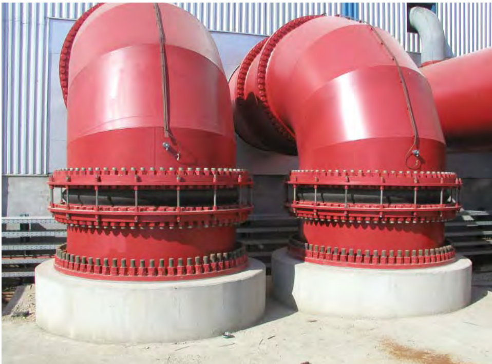
restraint compensator - design M DN 2600
