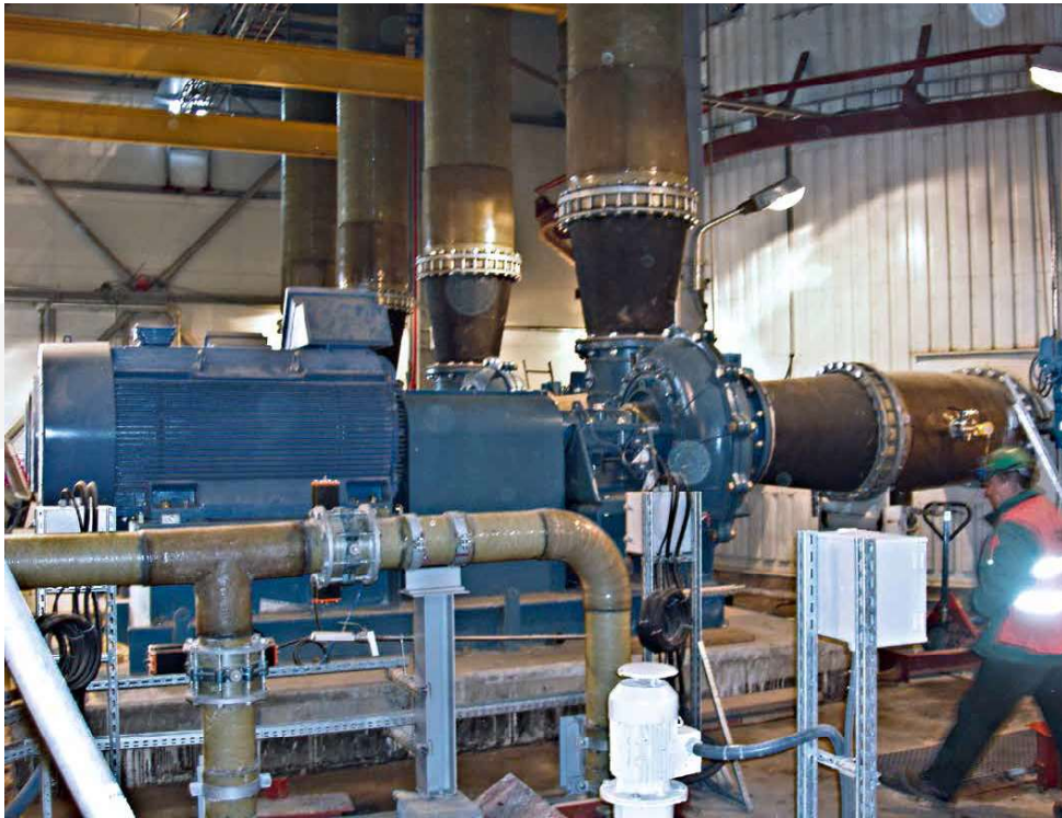
Conical expansion joints, type U300A on the suction and discharge side of a gypsum slurry pump in a desulphurization unit of a power plant
