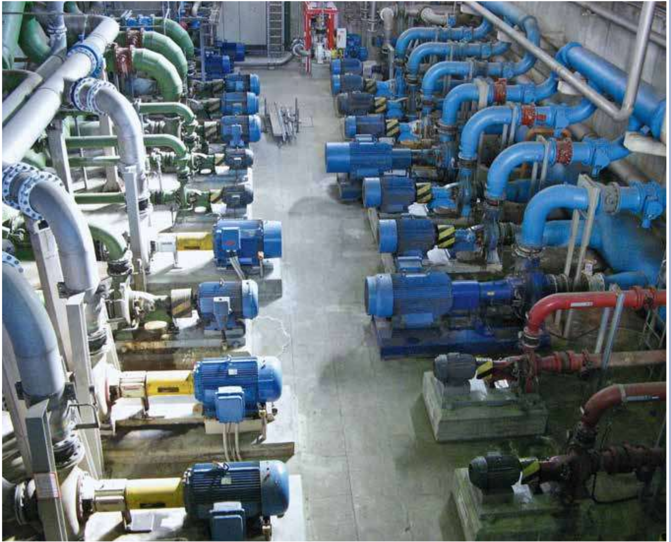
Universal expansion joint, type U110A on the supply pumps in a paper mill NB 80 – NB 350, 10 bar
