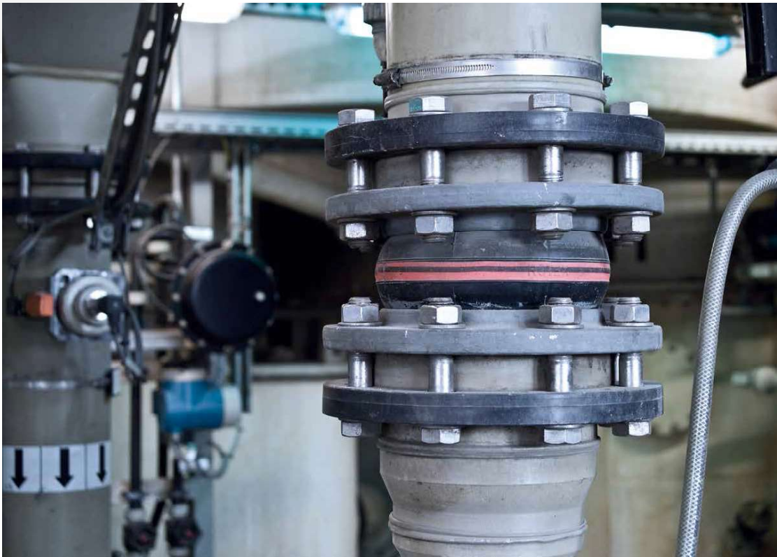
Universal expansion joint, type D110A in a plastic pipe of a paper plant NB 150, design pressure 6 bar
