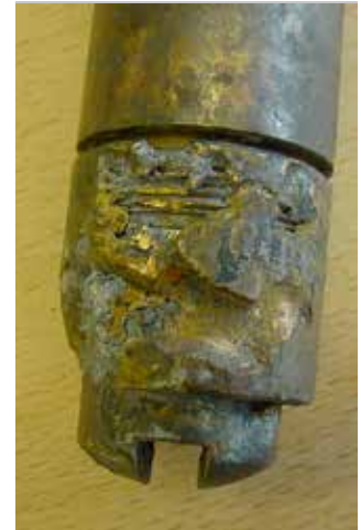
Mechanically worn retaining nut caused by roller contact. Nozzle extension pipe was not supported and aligned
